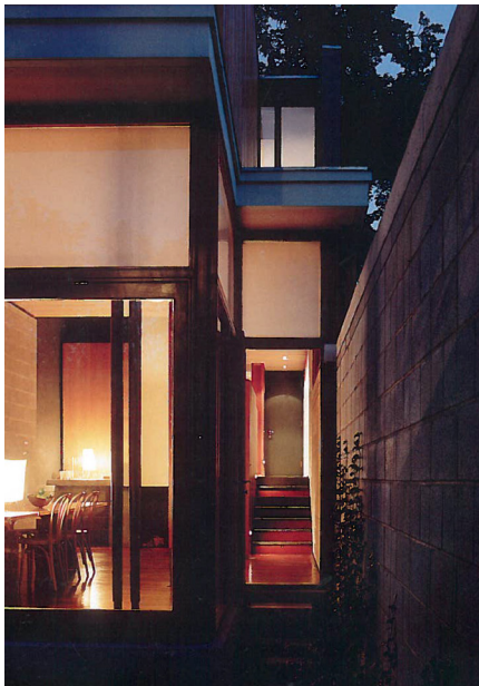
Right: Entryway to the Urban House by Shim Sutcliffe Below: Elevations and Section of the Urban House
